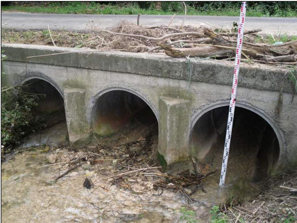
*PHOTO 27 : BUSES Ø1000 AU NIVEAU DU CHEMIN DES BAUX A MOURIES*
