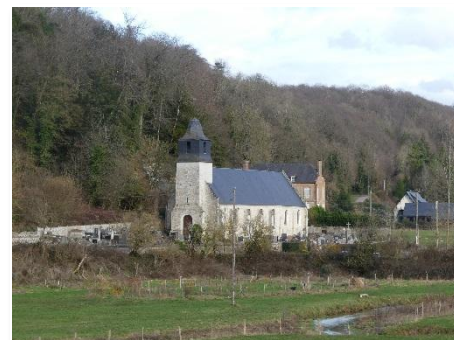
Centre village de Saint-Pierre-du-Val
