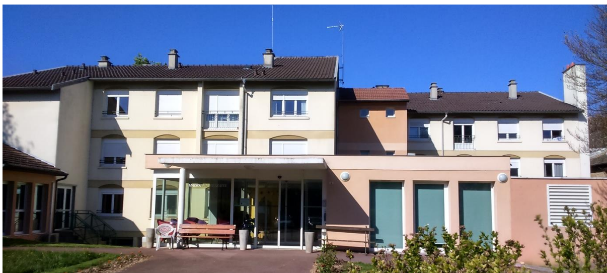
EHPAD de Saint-Gengoux-le-National
