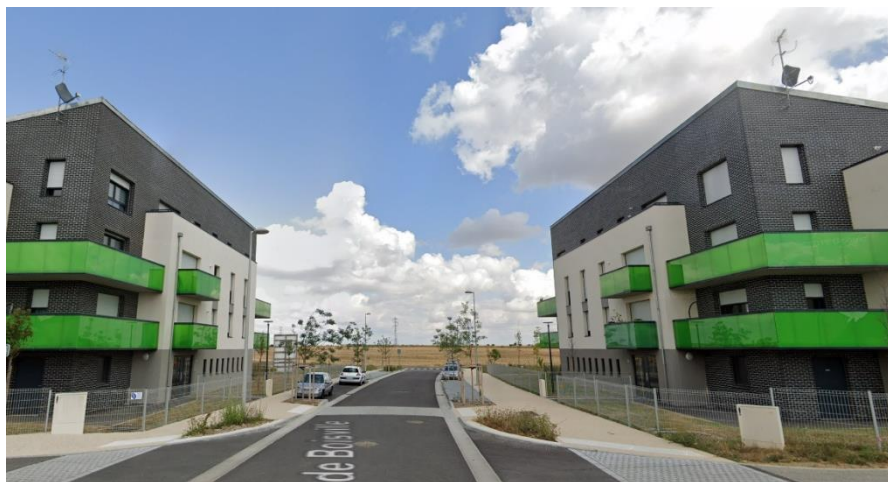
Figure 99 – Photo rue de Boisville - Source GoogleStreetMap –
