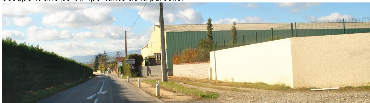
Hangar industriel imposant
