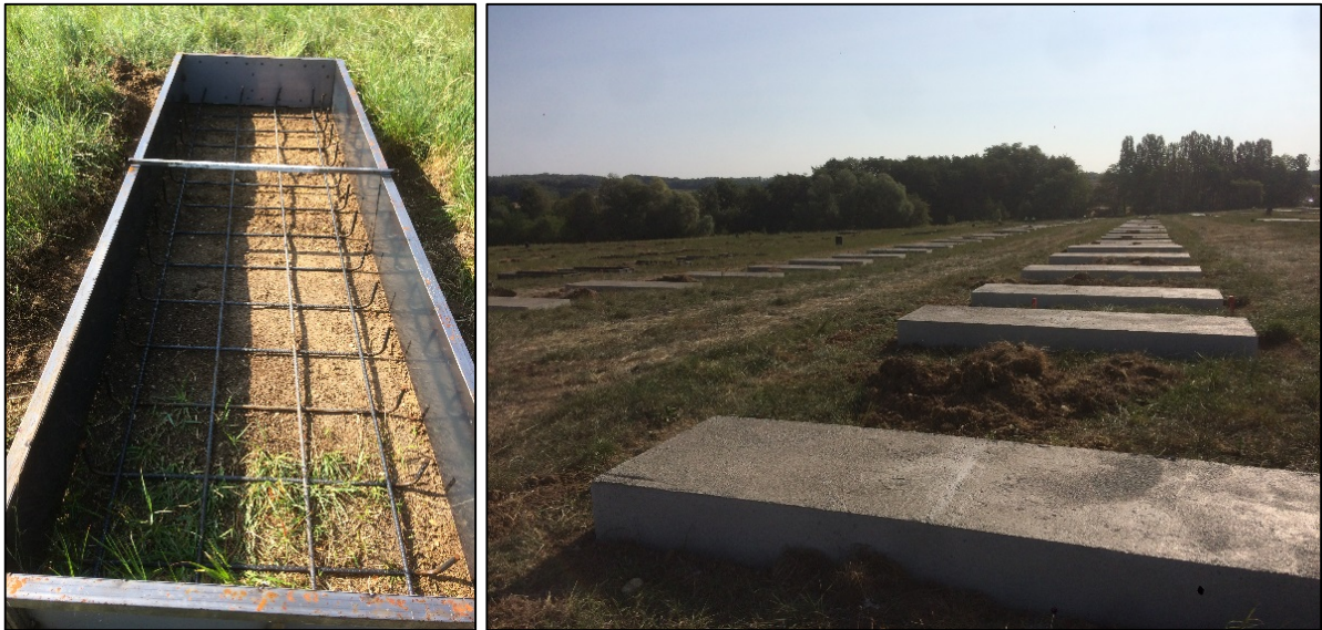
Photos de longrines, source ENGIE Green
