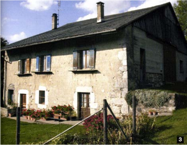
Ferme de village – bardage vertical - Le Bourgeau
