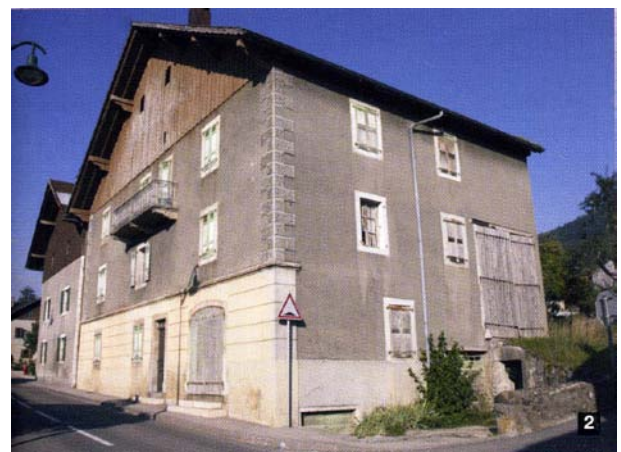
Maison de village – Bardage vertical - Villard
