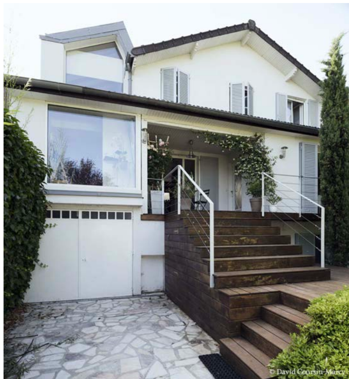
Extension maison ANGELES DUQUE - MIA ARCHITECTES
